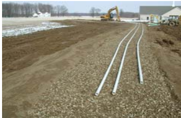
Experimental Mound Sewage Treatment System installation.
