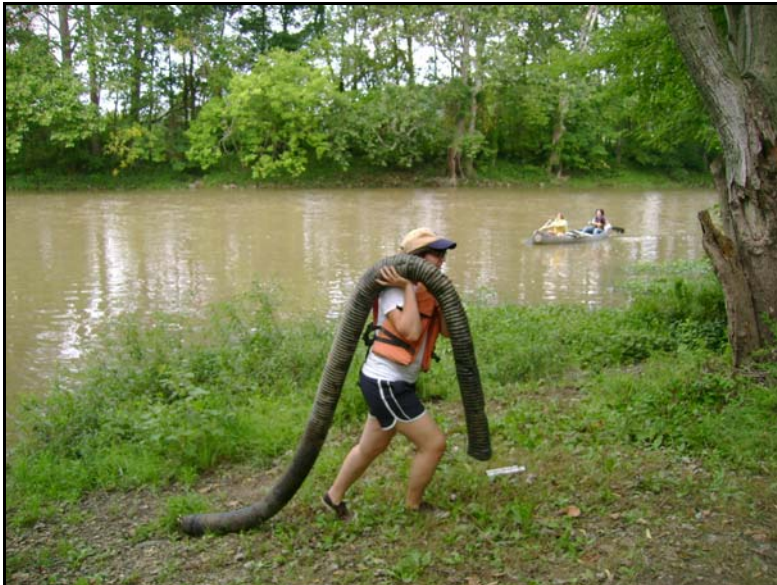
Ohio Wesleyan University student Maggie Argiro hauls a flexible drain pipe out of the Scioto River.
