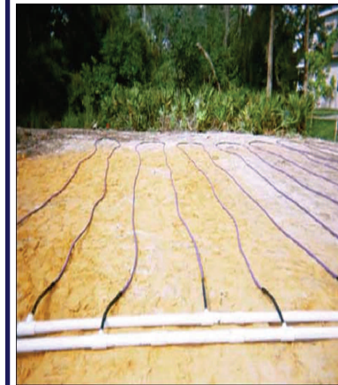
Layout of a Drip Distribution System
