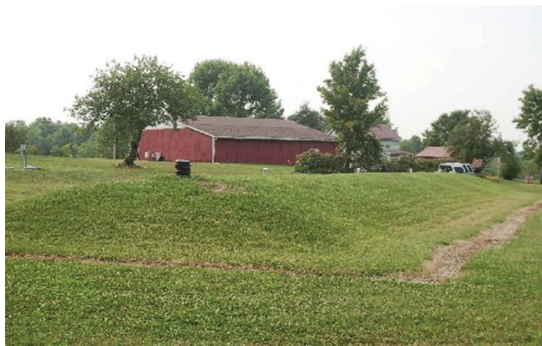
Finalized Mound System
