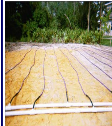
Layout of a Drip Distribution System
